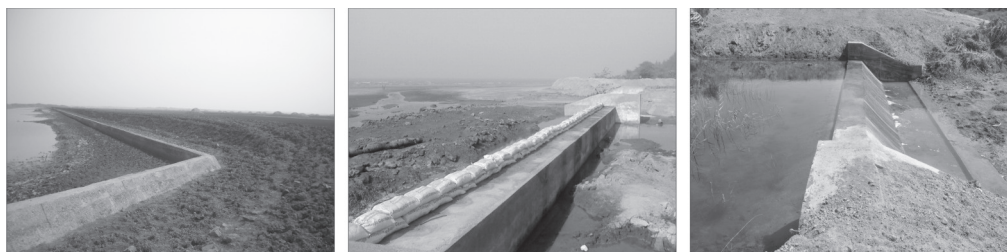
Fig. 1b. Physical structures to arrest sea ingress: Reclamation bunds (cement) and check
