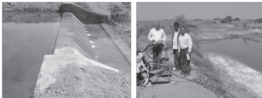
Fig. 5. Check dam (Kachhchh) and farm pond (Rajkot) with stored rain water during February-April period (onset of summer) provided irrigation water needs
