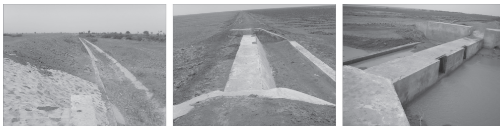
Fig. 1a. Physical structures to arrest sea ingress: Reclamation bunds (earthen) and check dams
